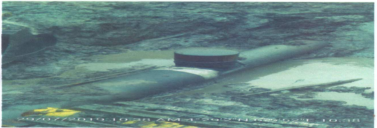
Repaired section during JIV
