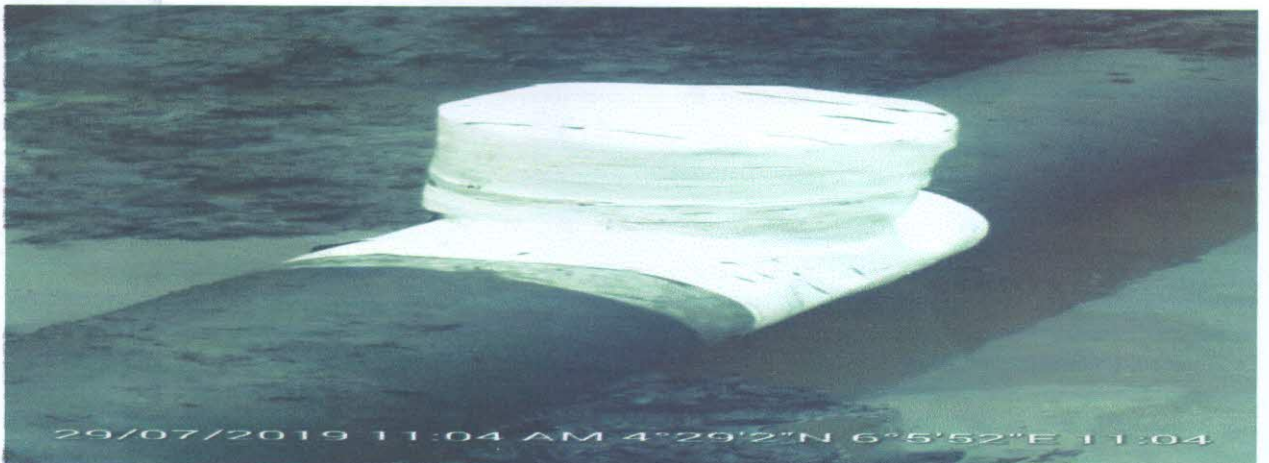
Completed section of the incident point.
